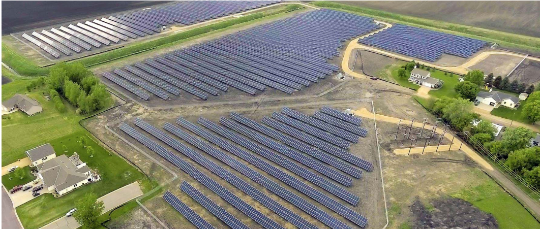
Mapleton, MN Solar Farm
